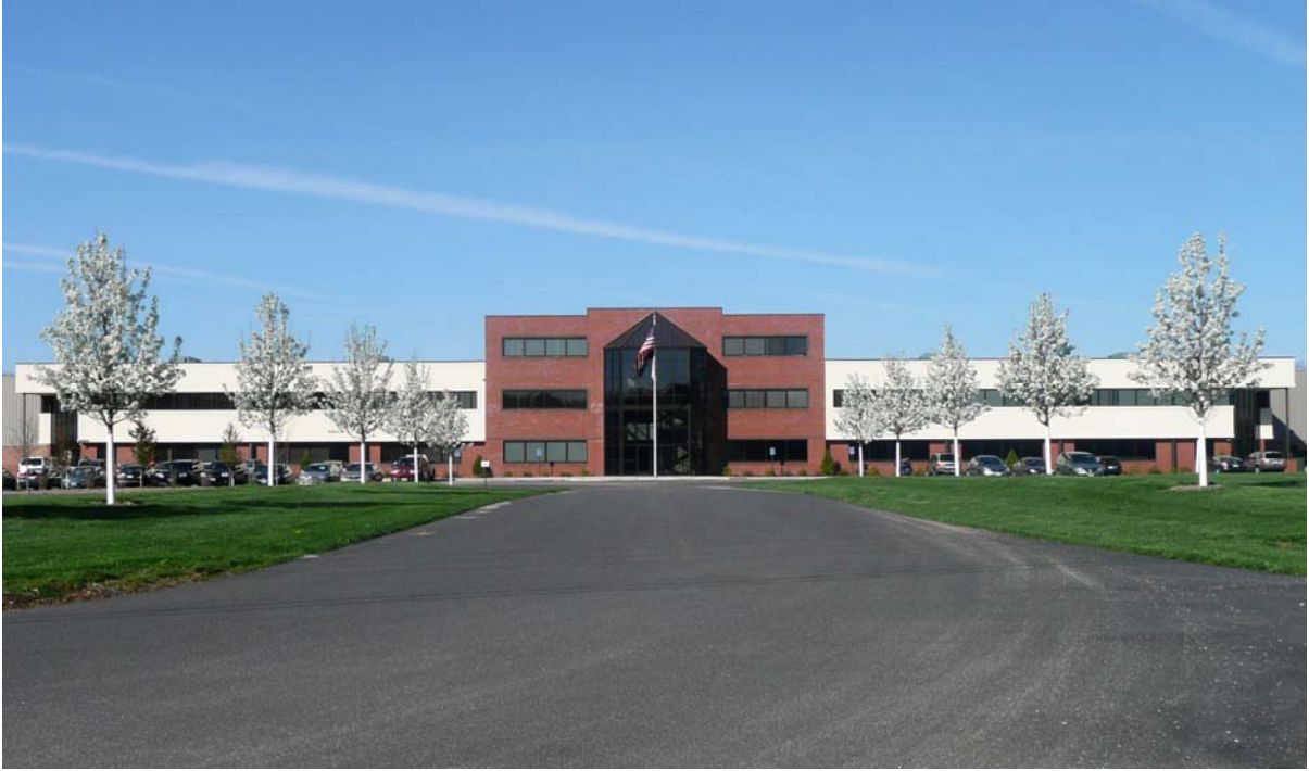
IQL Training Facility
