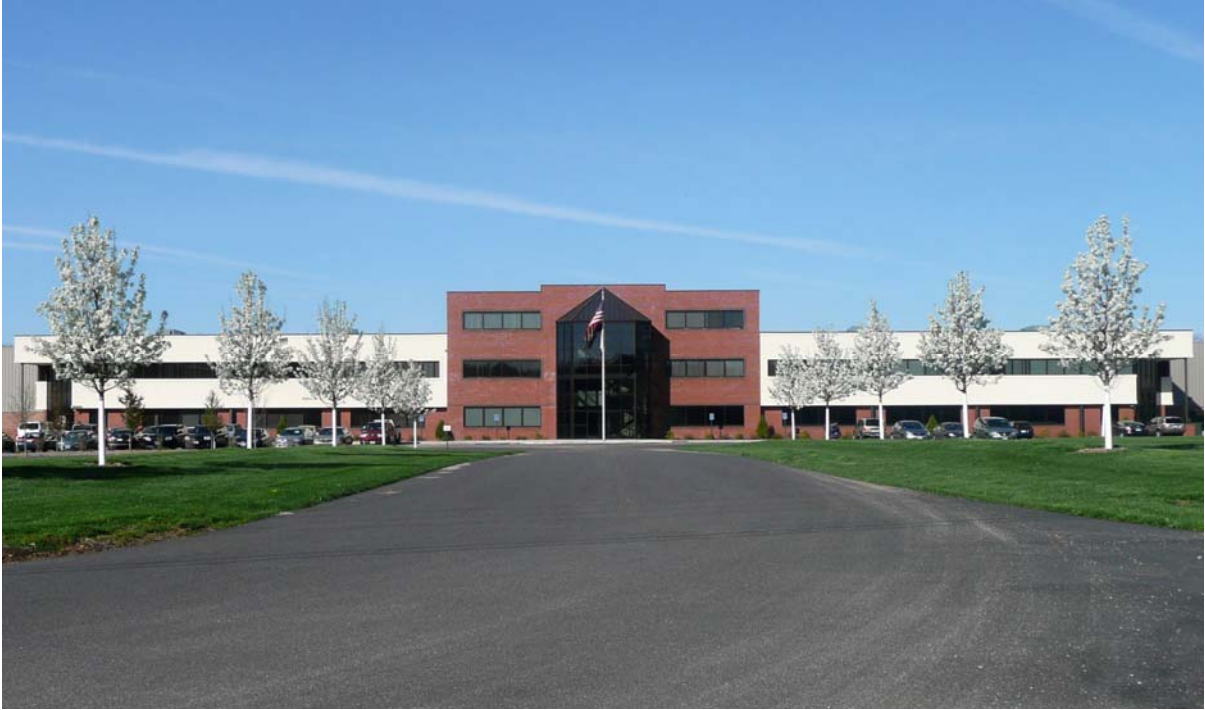
IQL Training Facility
